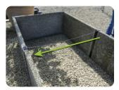
(9) Once your GreenBed<sup>™</sup> is square, add the wire cable to the center joiner brackets. Slip each end of the cable into the slot at the top of the bracket to provide additional strength.
