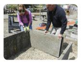
(7) Now install the end panel with the pre-installed corners (flush brackets UP!) to complete the walls of the bed. You will need to adjust the side walls to mate up with the corners of the end panel. Use the 1½" screws to secure the corners.
