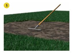
Level the garden site. This step is VERY IMPORTANT. If the site is level, installation will be MUCH FASTER. Remove rocks, roots and debris that may prevent the panels from sitting straight and level. Using a laser level to check your work can speed up this process. Compact the soil where the walls of the bed will rest.
